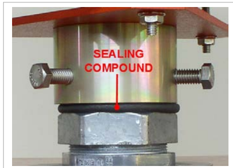
Figure 12 Co-mount Hub Sealing
